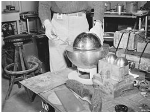
Slotin's assembly, Plutonium core hidden by Be reflector shells.
